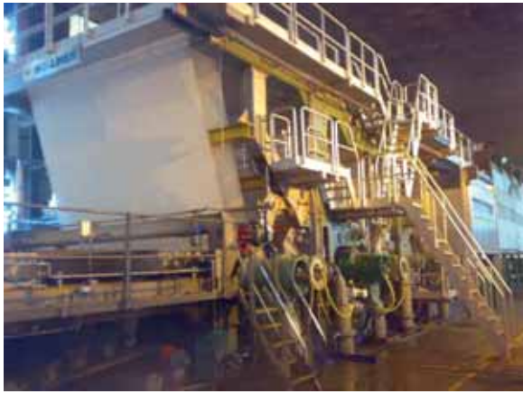
The new press section
