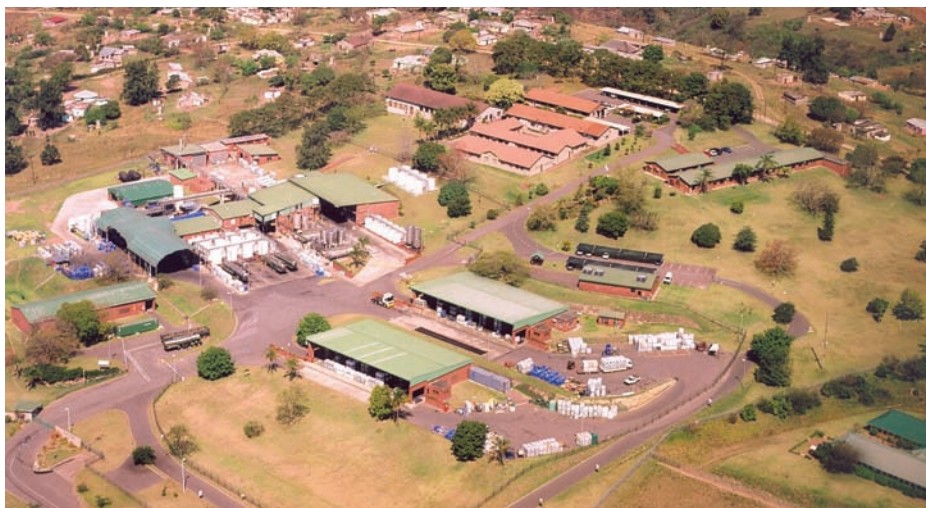
FROM THEN 'TIL NOW: The Buckman Laboratories premises in Jacobs, 1973 (far left), was followed by a more expansive plant in Hammarsdale. Early construction in 1978 (middle) on the plant has culminated in the current Buckman Africa plant (left).
